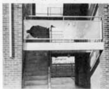
31 Completed glass, judiciously framed in steel
